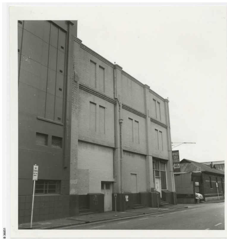
State Library of South Australia - Wyatt Street [B 36851], Wyatt Street, east side, right side of building is 41 yards north of Flinders Street and frontage is 18 yards. 1979. Photographer, State Library of South Australia, Part of Acre 231 Collection.
